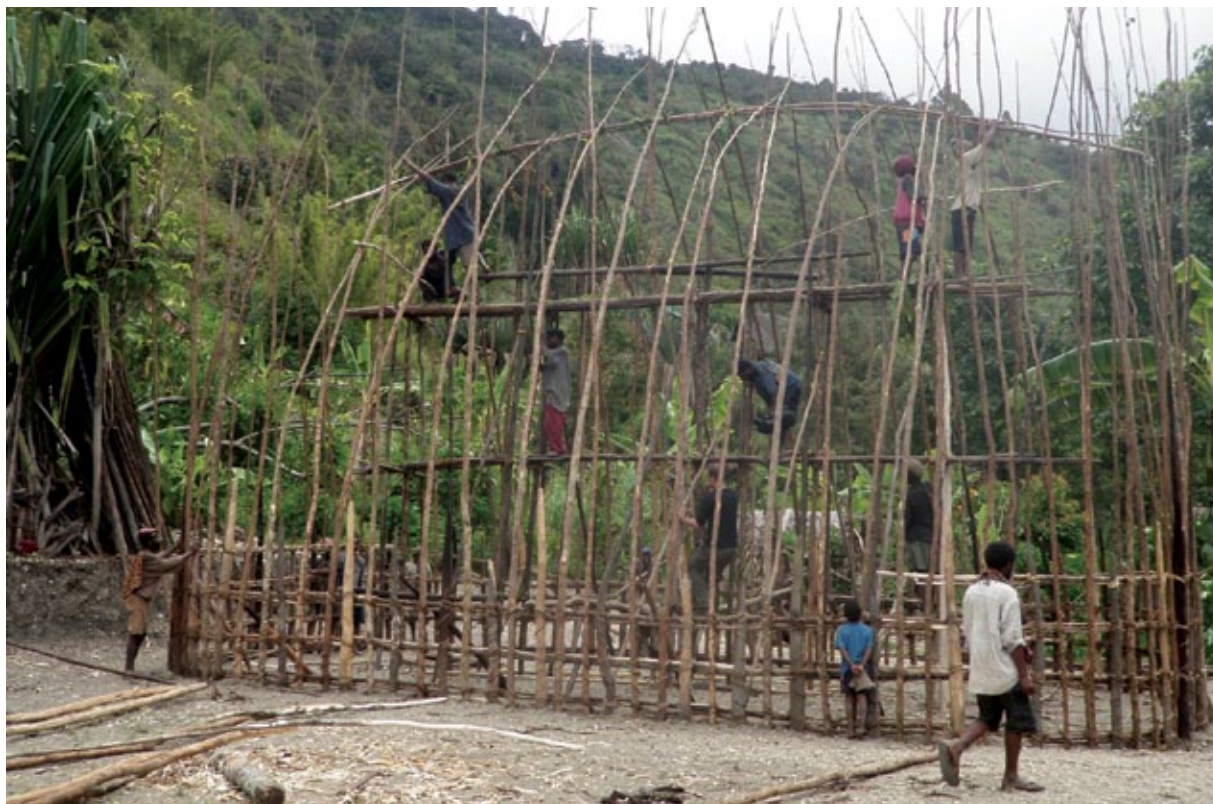
Constructing a traditional house from bush materials in Teptep village
