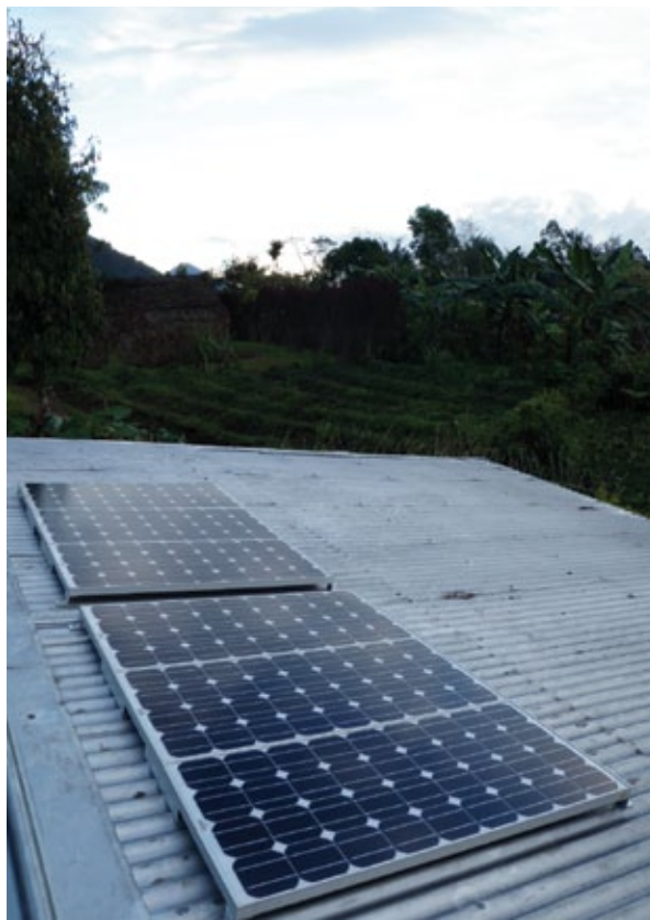
Solar panels for Bungawat solar fridge
